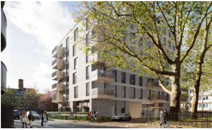
View along Grant Road, Block A
